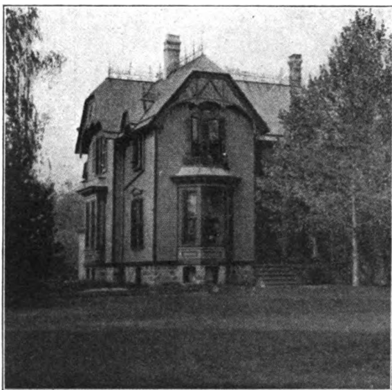
Dwelling No. 2 Faculty Row. No. 3 is same style, built 1874.
